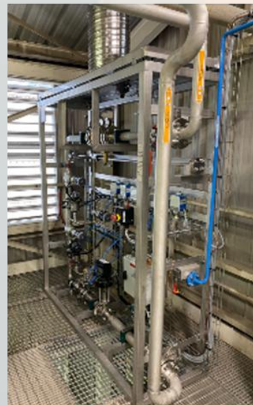
Safety and regulation skid H2
