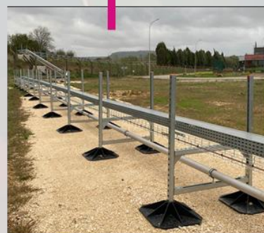
H2 piping @ 10 bars length ~500m
