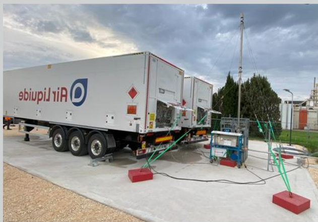
H2 decompression platform 300 bars => 10 bars
